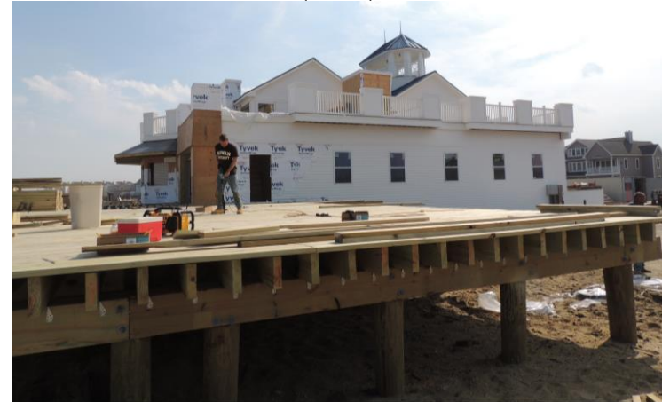
Figure 38: Repairs to the Bathing Pavilion on May 16, 2013 (1 of 2)
