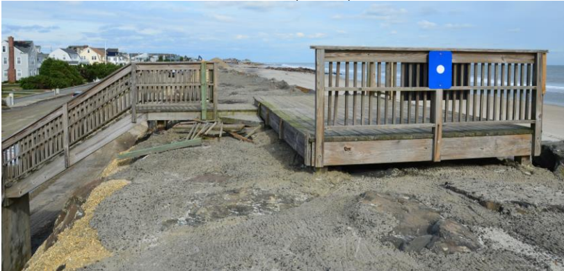
Figure 19: Damage to the Public Access Stairs at Seacrest Avenue
