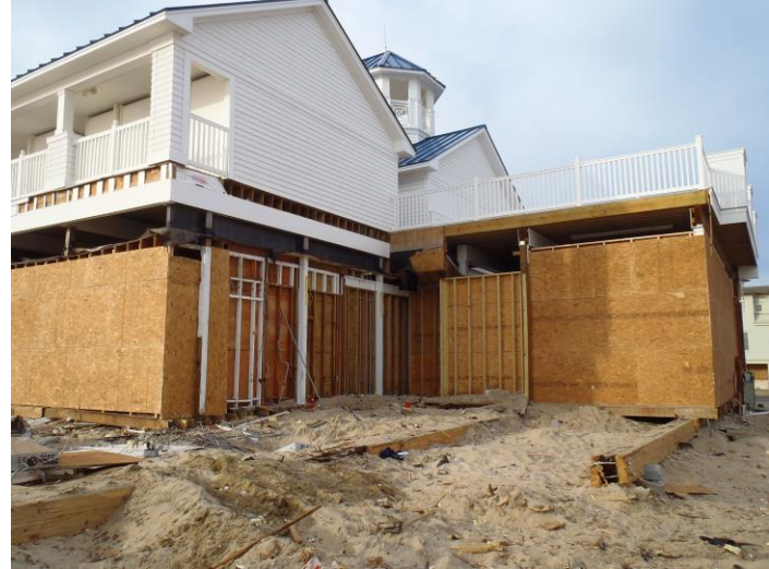
Figure 29: Damage to the Bathing Pavilion (6 of 8)
