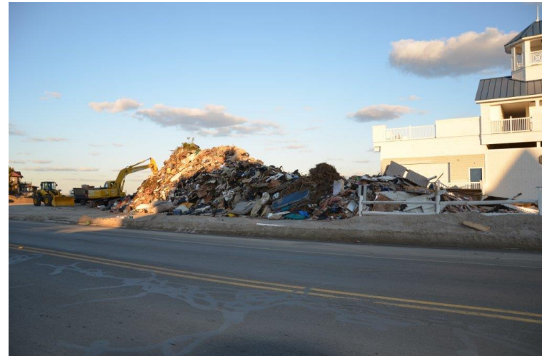
Figure 32: Debris is temporarily placed at the Bathing Pavilion.
