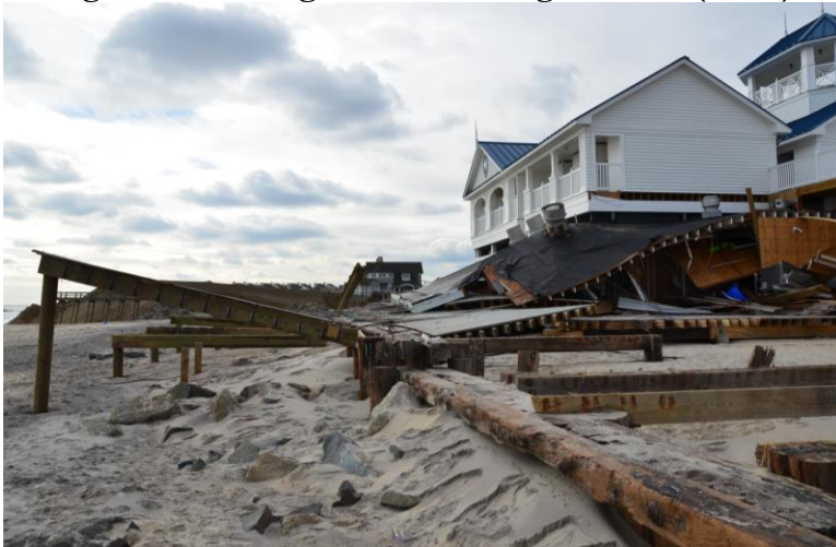
Figure 24: Damage to the Bathing Pavilion (1 of 8)
