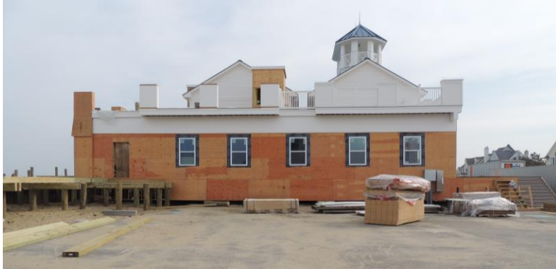
Figure 37: Repairs to the Bathing Pavilion on May 10, 2013
