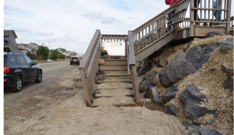
Figure 21: Damage to the Public Access Stairs near Seacrest Road before They Were Removed and Relocated
